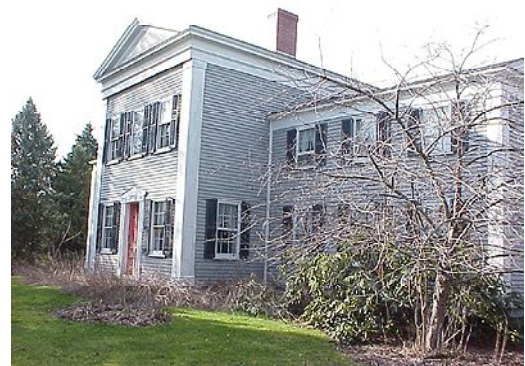
Site Photo: Clarke Home
