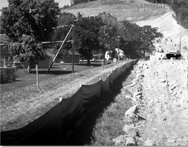
*A silt fence is an effective practice for controlling construction site erosion/sedimentation if properly installed and maintained.*
